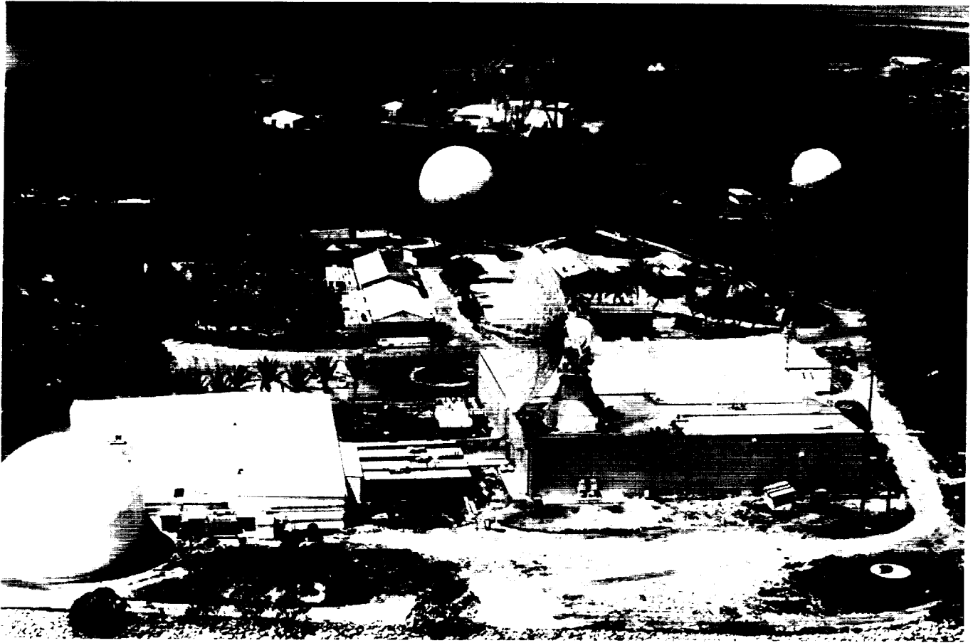
Photograph of the Kiernan Reentry Measurement Site located on Kwajalein Atoll. The site has four radars which operate at six separate wavelengths ranging from 193 to 1 cm.
